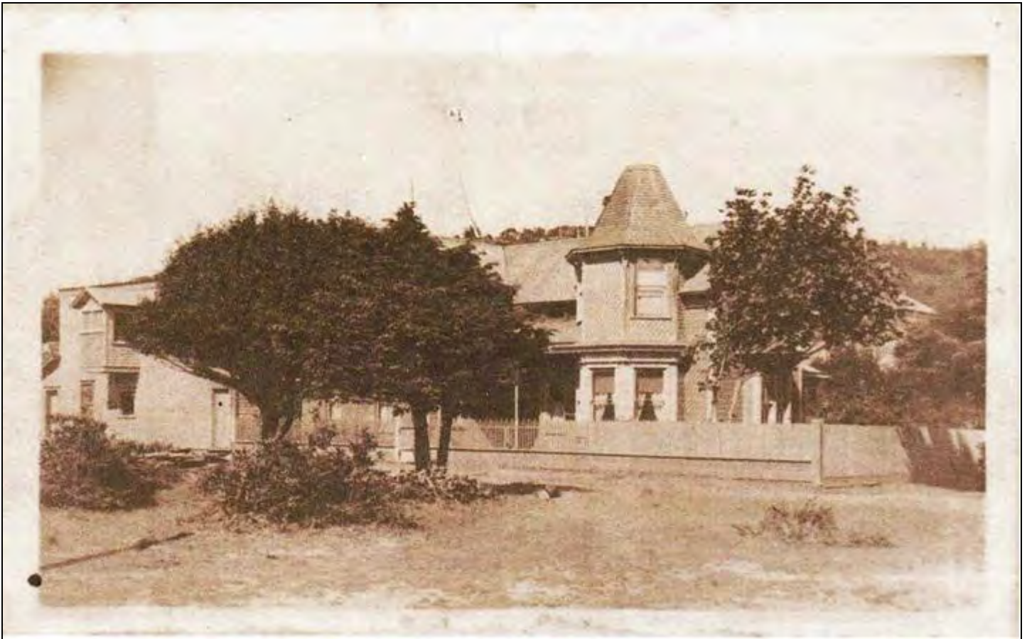
Figure 9: Peter John Lindberg House (c.1910), earliest known picture of the house, looking northeast.
